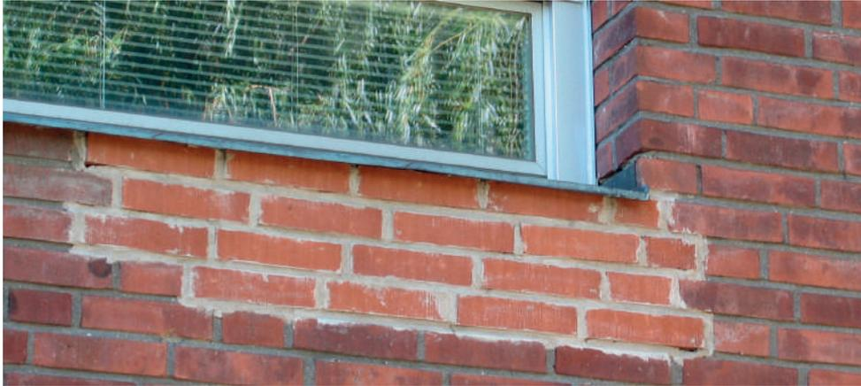
Figure 2. An example of adverse effects of selecting unsuitable mortar and shoddy workmanship on repointing
